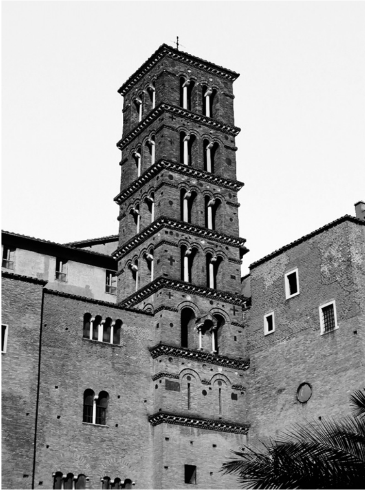
Figure 3.2.6. Romanesque church tower, from the late 1300s. Rome, Italy.
