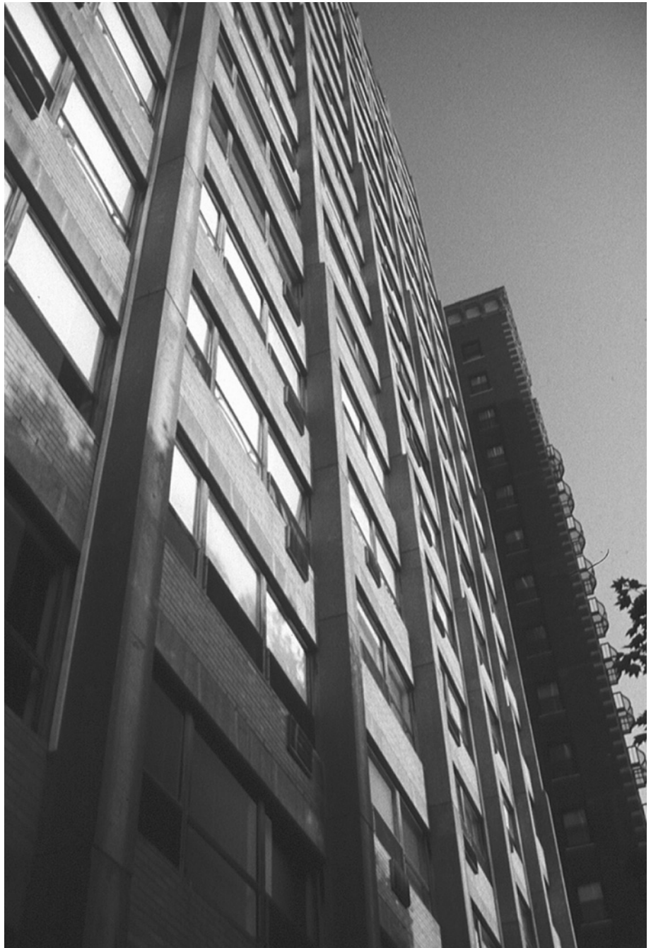
Figure 4.5.6. Columns showing the additive effects of multiple floors. As the tributary load increases, the columns step out toward the building’s base, reflecting the need for greater cross-sectional area. (Note that stepping out in one direction does nothing to increase the column’s slenderness ratio, which isn’t always a problem with short story heights). Promontory Apartments, Chicago. Mies van der Rohe, Architect; Frank Kornacker, Engineer.
