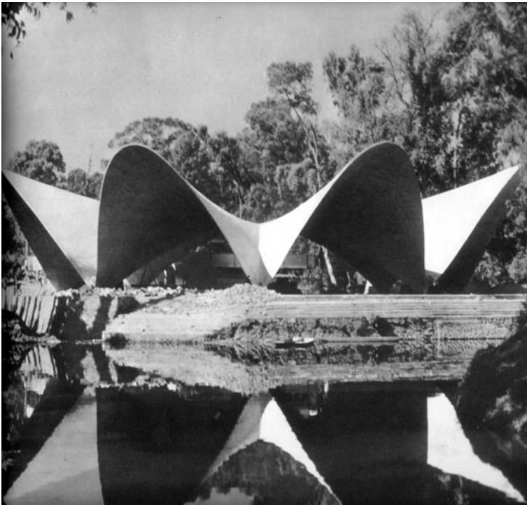
Figure 3.5.7. Thin shell concrete structure, restaurant, Xochimilco, 1958.
