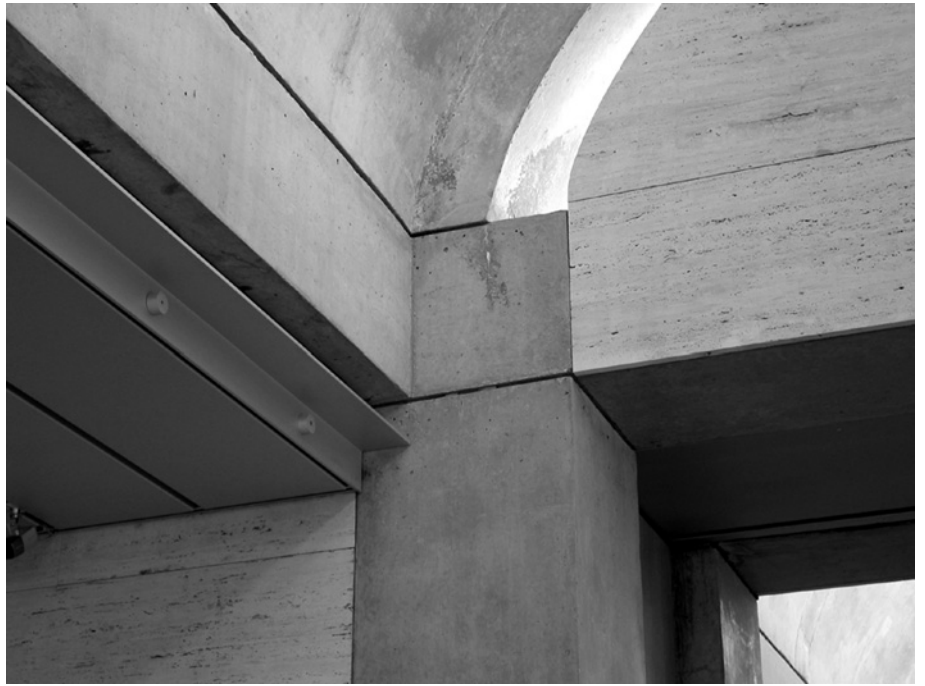
Figure 5.5.9. In contrast to Mies' Farnsworth House, Louis Kahn's Kimbell Art Museum in ort Worth, TX, adopted an intensive program of expression, with pour lines in concrete detailed to show just how its pours were sequences. Aluminum and travertine finishes were attached with reveals and shadow lines to show that they were clearly assembled after the concrete frame.
