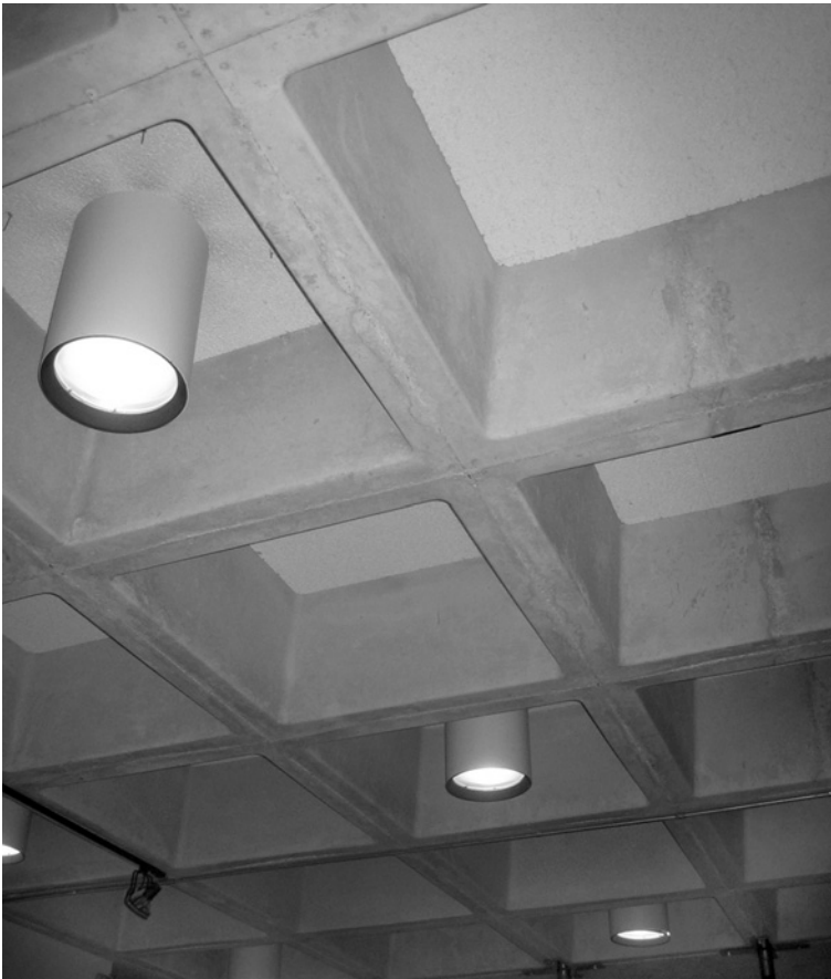
Figure 4.6.6. A typical two-way ('waffle') slab.
