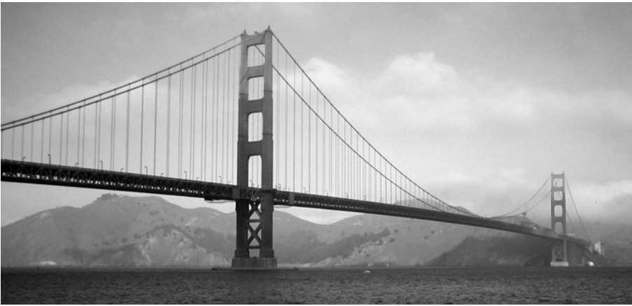
Figure 4.2.14. Perhaps the most famous funicular of all, the cables of the Golden Gate Bridge (and all other suspension bridges) are pure catenary shapes, reflecting the additive loading of the bridge deck (a distributed load) being transferred through pure tension elements to the towers.
