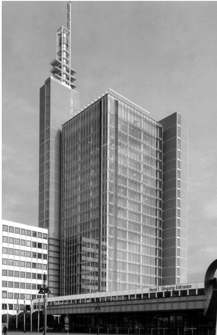
Figure 5.2.14. Double skins offer visual depth and a refined texture, in addition to their environmental benefits. (World Trade Tower, Hannover Thomas Herzog, 1998)
