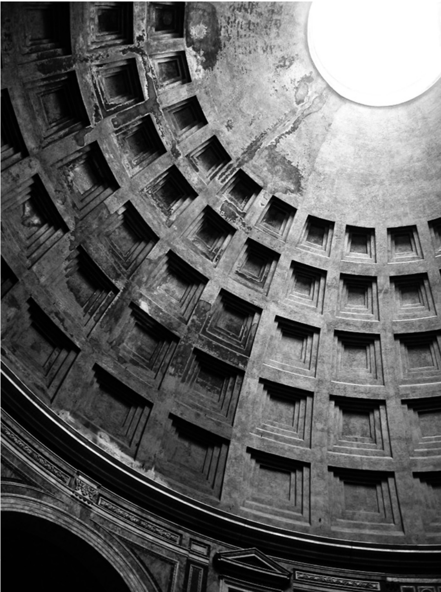
Figure 3.5.3. Pantheon dome, 118–126, Rome, Italy. The coffered concrete dome spans 40 m.
