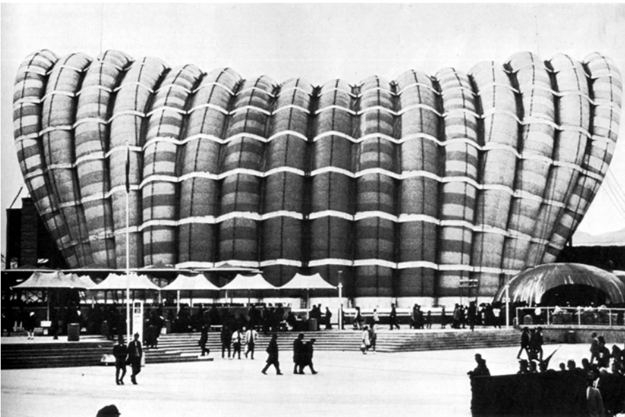
Figure 4.9.14. A pneumatic structure (Fuji Pavilion, Osaka EXPO 1970) that used pressurized tubes to avoid the need for complicated revolving doors and pressure maintenance devices.
