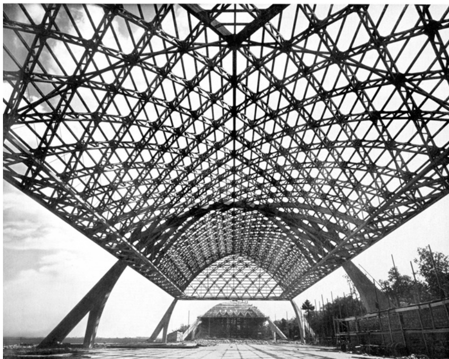
Figure 3.5.6. Pre-cast airplane hanger structure, 1940s, Pier Luigi Nervi. Italy.
