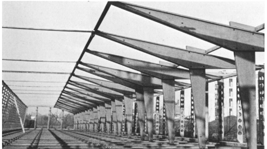
Figure 4.3.19. Beam design often mimics the shape of moment diagrams to distribute material where it will do the most work. Here, a prototype school by Jean Prouve (1954) uses ideal cantilever shapes; deep at the root, tapering toward the tip, reflecting its shear and moment diagram (see Fig. 4.3.17). (From Benedikt Huber and Jean-Claude Steinegger, Jean Prouve).
