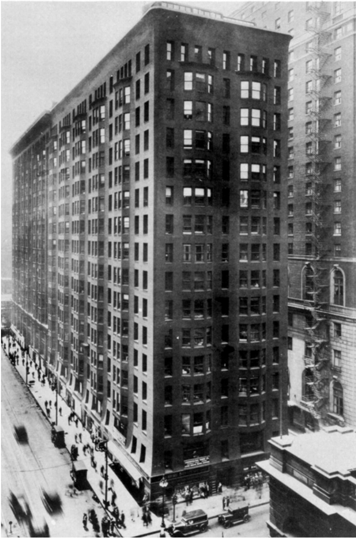
Figure 3.2.8. Monadnock building, 1889–1891, Chicago, Illinois by Burnham and Root. The classic brick load-bearing skyscraper. Sixteen floors tall.
