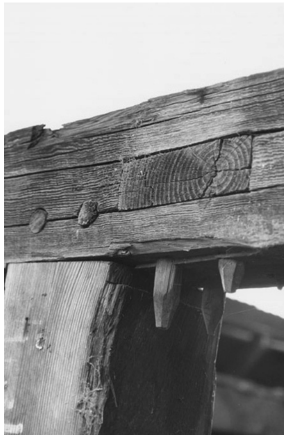
Figure 3.1.7. Barn heavy timber joint, from the late 1800s.
