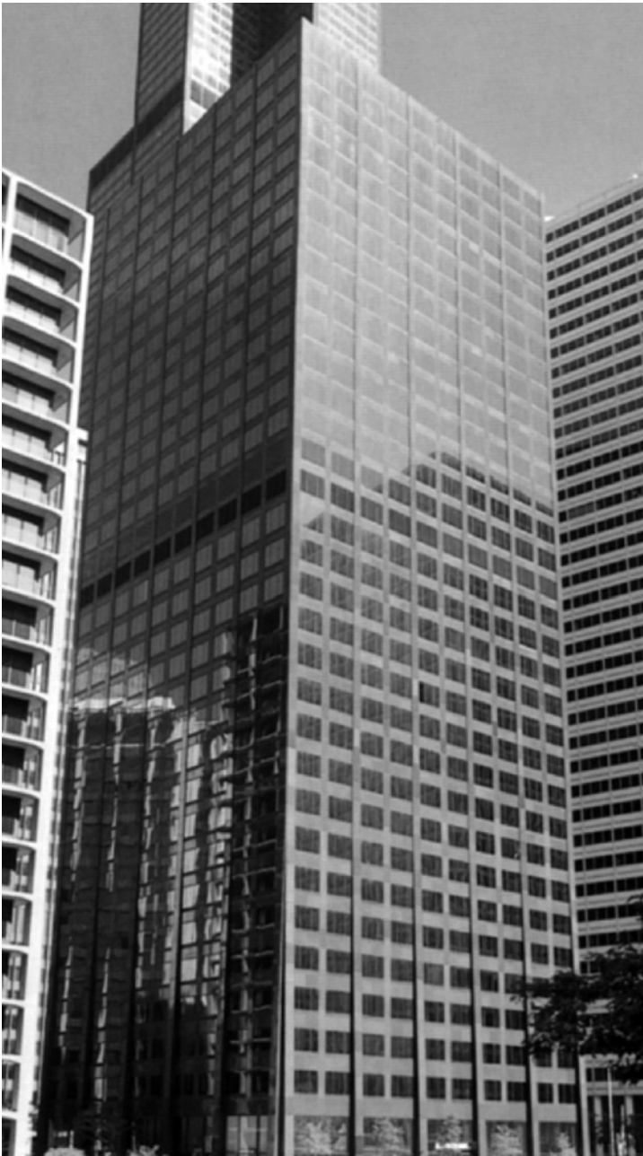
Figure 4.5.7. Column theory as architectural expression. Note the gradual thickening of columns toward the base, and the use of intermediate tension columns to support the second floor, opening up the ground floor. Riverside Plaza, Chicago. Bruce Graham/SOM, Architect; Fazlur Khan/SOM, Engineer.
