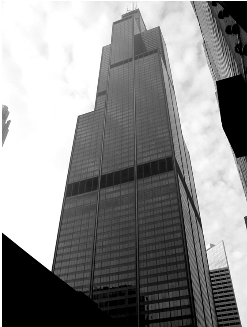
Figure 4.8.10. Chicago architecture of the post-war area contains numerous examples of the frame used as architectural device. The Sears Tower (Bruce Graham and Fazlur Khan of SOM, 1961) uses moment frames bundled into nine tubes, essentially super-scale columns with the majority of their stiffness on their perimeter.
