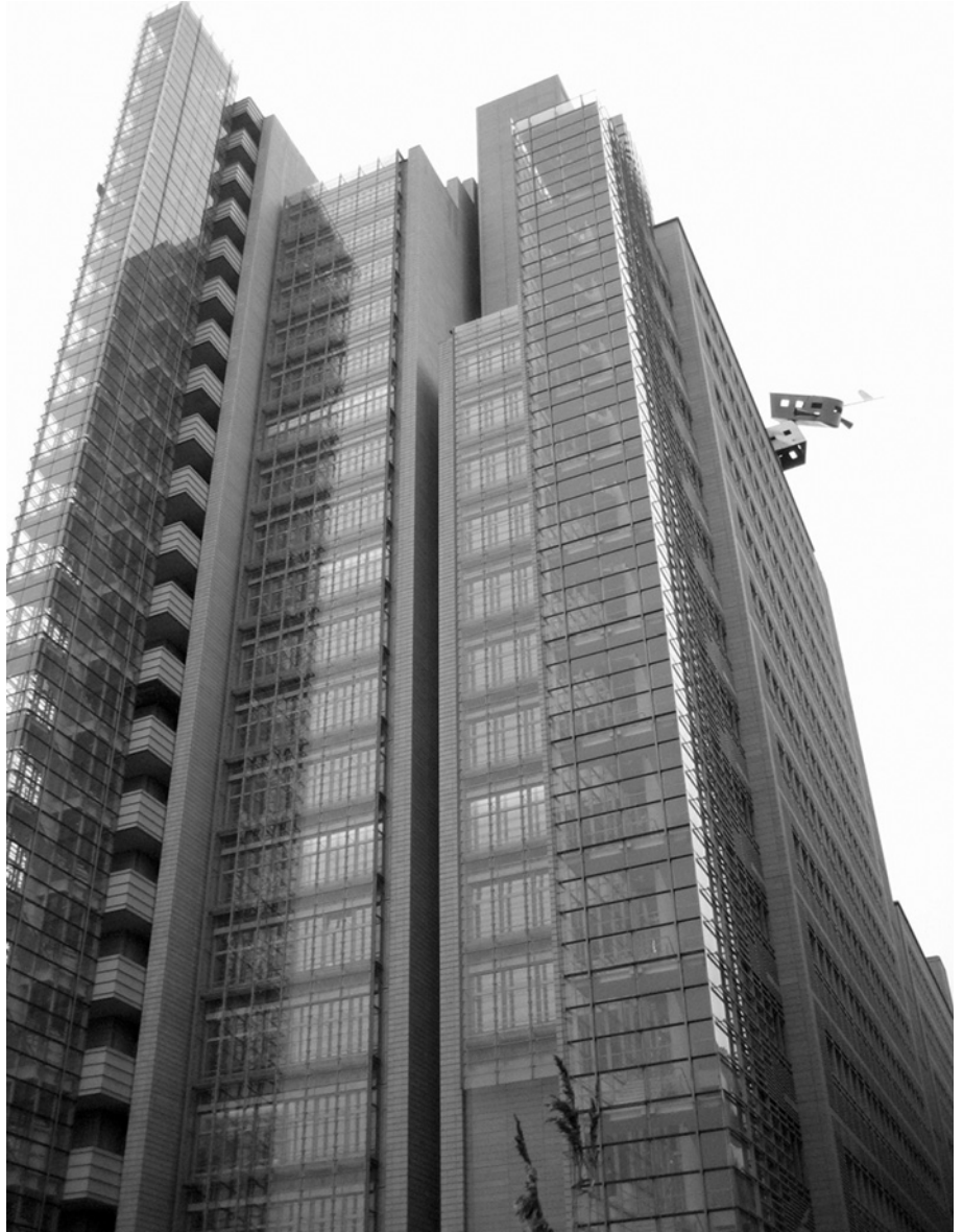
Figure 2.1.10. The fire stair as architectural element. Renzo Piano's Debris Building in Berlin uses fire stairs to articulate its end facades. Because containment requirements only apply to walls between occupied areas and the stair tower, most codes permit glass enclosures for stair walls that are not contiguous with spaces that may burn (there may be restrictions on how close the glass can be to an opening in the building wall, however). Since stairs relate both the horizontal grain of a building (its floor levels) and size of its occupants (the treads, risers, and handrails), they can provide a sense of building and human scale.
