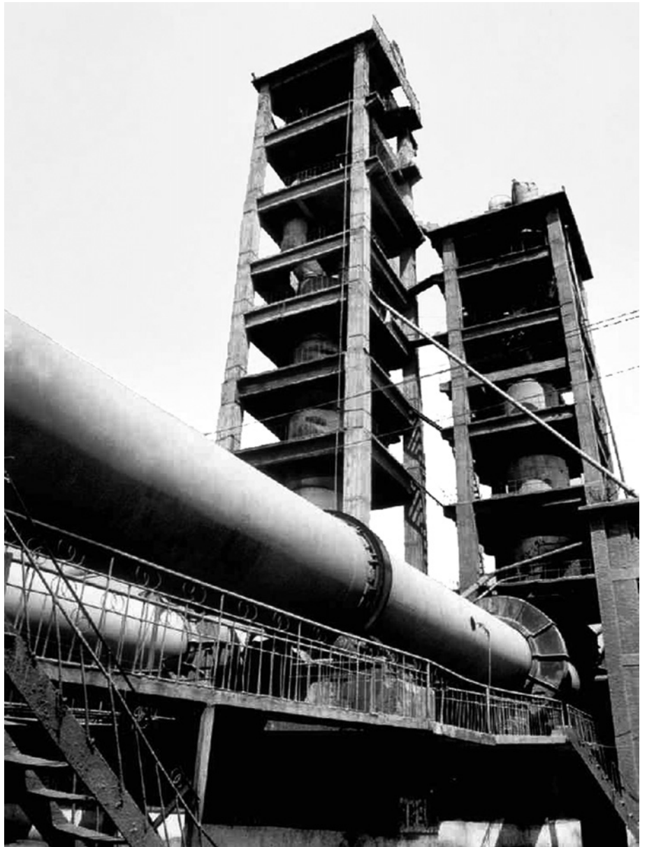
Figure 3.5.2. Rotary cement kiln.
