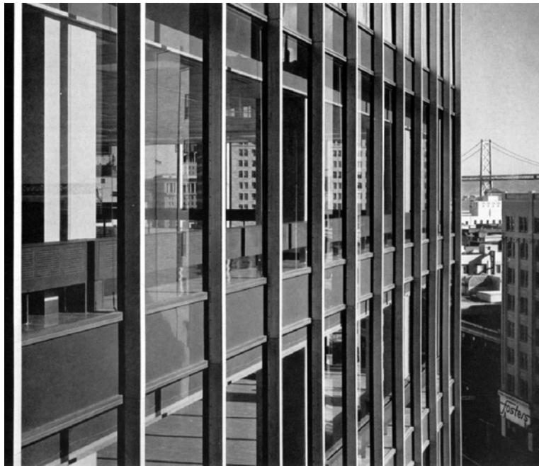
Figure 5.2.10. A metal and glass curtain wall from the 1950s that remains a particularly elegant example; the Crown Zellerbach Building in San Francisco.
