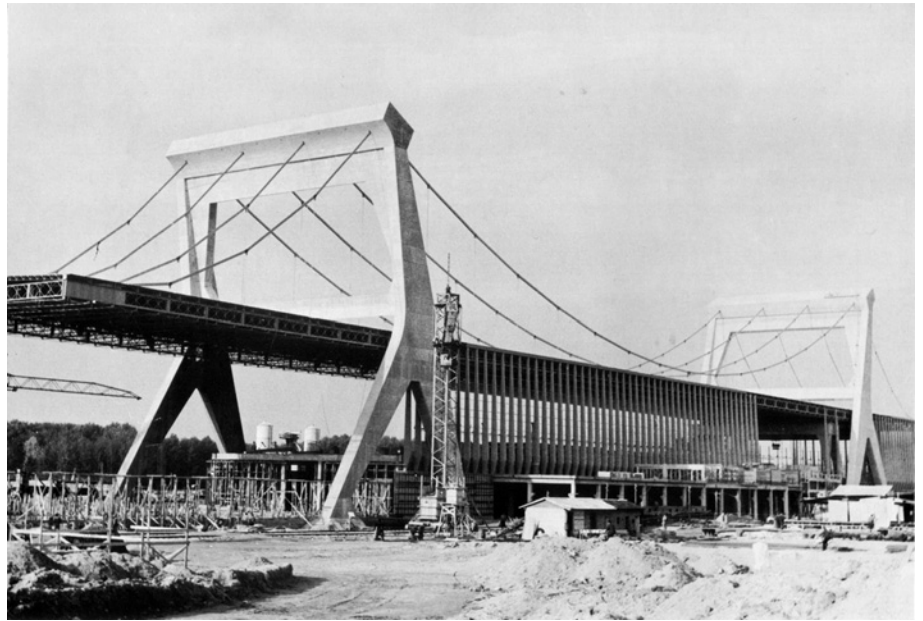
Figure 4.9.12. A rare example of a architectural suspension structure, the Burgo Paper Mill by Nervi. In this case, the roof might have been more efficiently carried by a more traditional system, but the result is a clear statement of the complex forces at work in a suspension structure – note the towers ‘lean’ that helps counteract the tendency of the cables to pull them toward one another.
