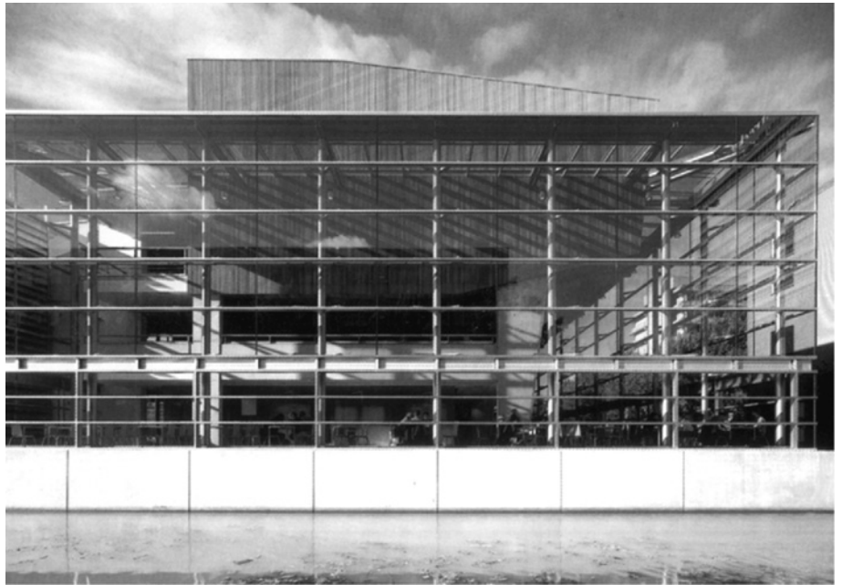
Figure 5.2.4. A typical (though thoughtfully composed) glass curtain wall.
