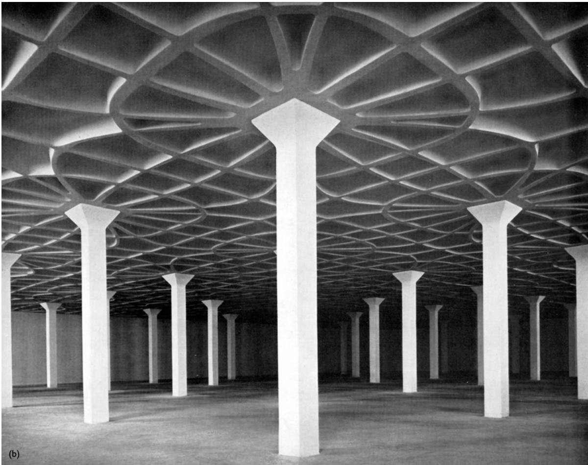
Figure 4.6.7. An experimental concrete floor system designed by Pier Luigi Nervi for the Gatti Wool Factory in Rome (1953). By using custom-shaped pans (of light cement and wire), Nervi was able to re-configure a standard waffle slab so that its ribs followed the lines of static 'flow' from slab to column.
