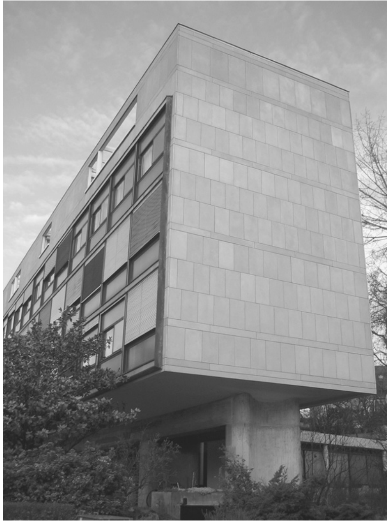
Figure 5.5.12. Corbusier's Swiss Pavilion at the Cite Universitaire in Paris blends glass, concrete, stone, and metal into a rich pattern that has both regularity and variety. The cladding is set just outboard of the solid wall, again telling us something about how the building was assembled and how it works. The end wall is plain, but it isn't inarticulate – the pattern of stonework describes the building section by revealing the floor locations. Finally, while the building could have been held up by a simple pier, the curvilinear shape at the base actually tells us – subtly – about the building's lateral stability, with two 'flanges' at the outer edges in the short (therefore weaker) direction of the building above.
