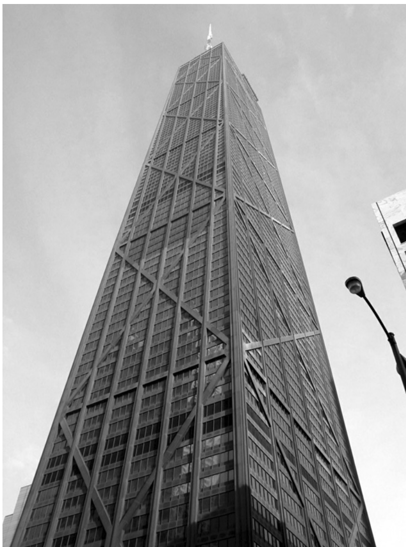
Figure 4.8.11. The John Hancock Tower (Bruce Graham and Fazlur Khan of SOM) uses cross bracing for both its lateral stability and its gravity system, lightening its total weight considerably.
