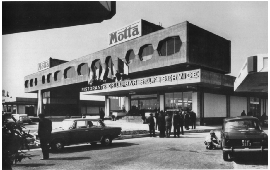
Figure 4.4.8. Structural design often takes advantage of the neutral axis to eliminate material from the center ‘web’ of beams. Here, a motorway restaurant by Pier Luigi Nervi replaces much of its concrete beam’s ‘web’ with window glass.
