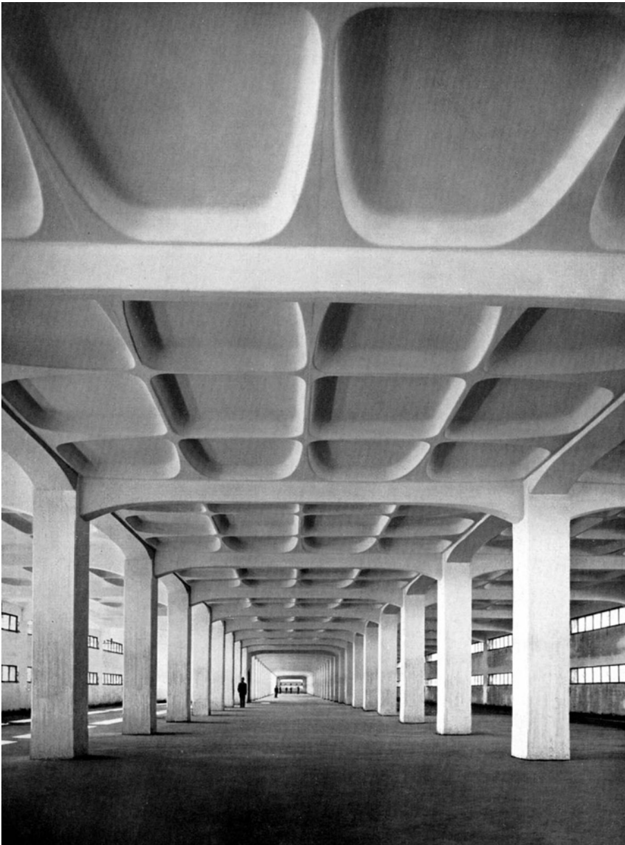
Figure 4.6.8. Another expressive floor slab by Nervi. This one, for a tobacco factory in Bologna (1952) thickens the ribs of a waffle slab where they meet supporting beams – and where they experience the greatest shear stress.
