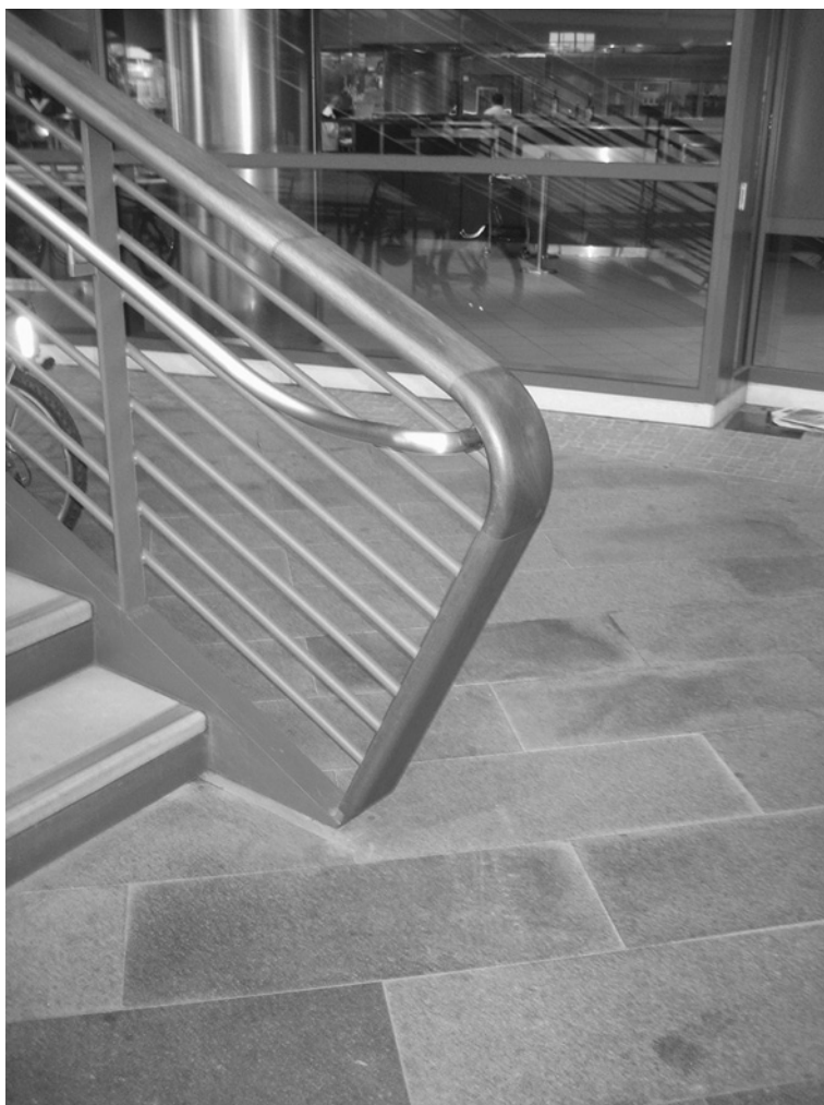
Figure 2.3.9. A carefully thought out arrangement of handrail and guardrail that offers gripping surface well past the final tread and fall protection without sacrificing aesthetics. (Clark Center, Stanford University. Foster and Partners.)
