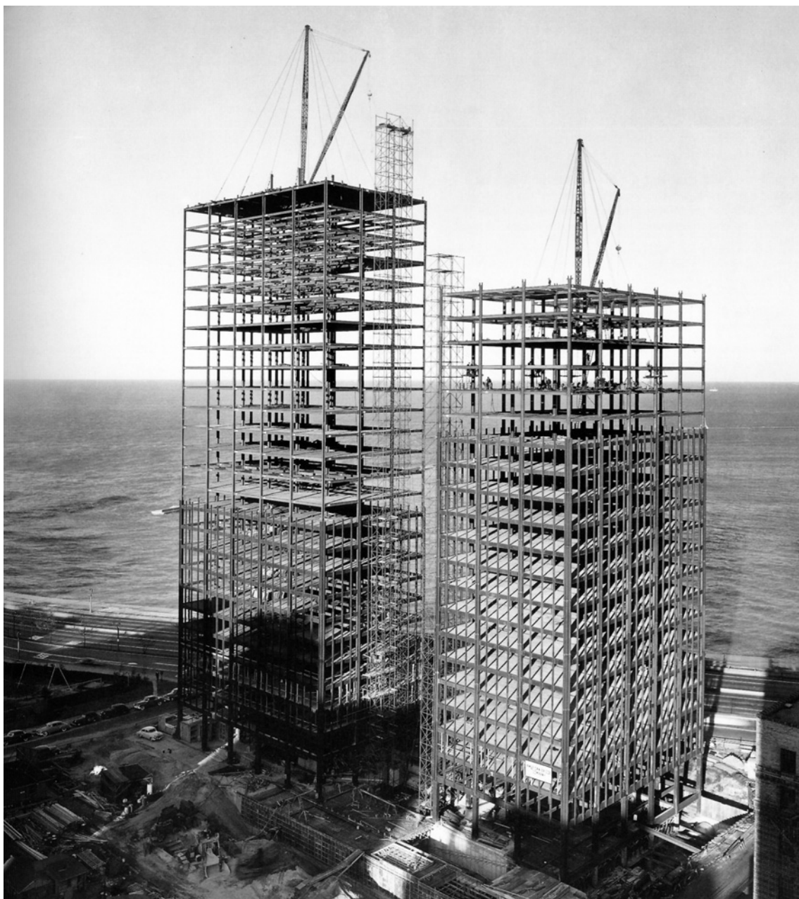
Figure 4.8.1. The structural frame has been one of the defining architectural expressions of high-rise construction. Mies van der Rohe's Lake Shore Drive Apartments (1949) pioneered the frame as a compositional element.
